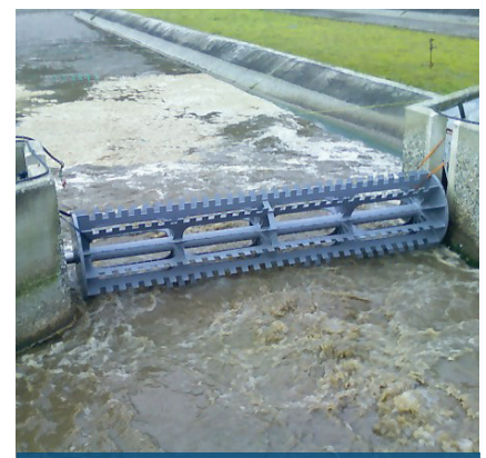
Aerator protected with Belzona coating
