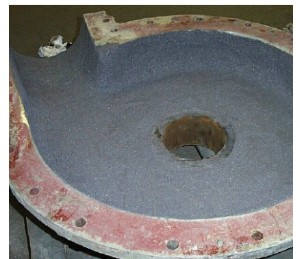
Abrasion resistant coating applied
