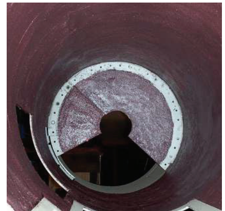
Rebuilt and protected against abrasion
