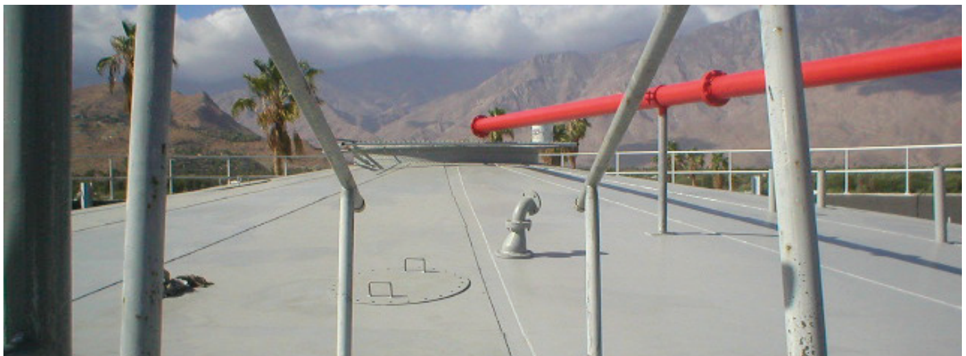
Tank roof restored with a Belzona protective coating
