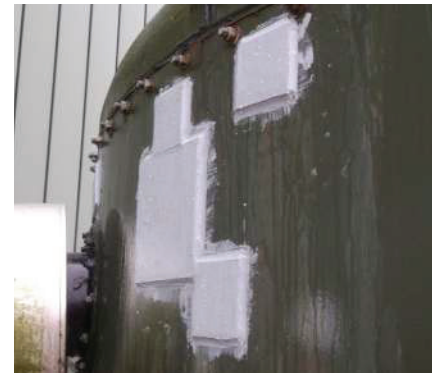
Tank repaired by cold bonding
