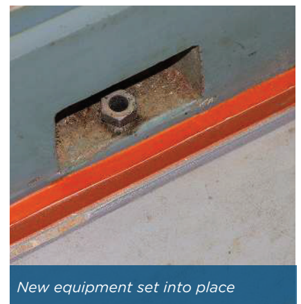
Belzona 100% solids chocking compound applied
