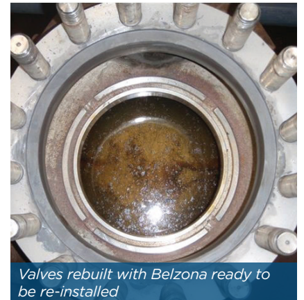
Internal surfaces rebuilt and protected with Belzona coating
