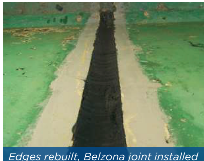
Edges rebuilt, Belzona joint installed
