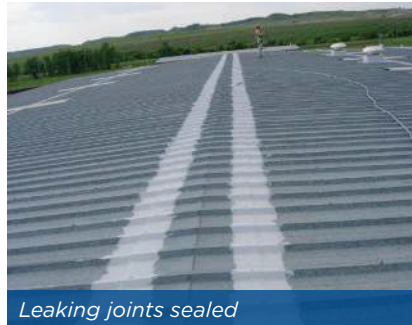
Full roof encapsulation
