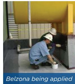
Concrete rebuilt
