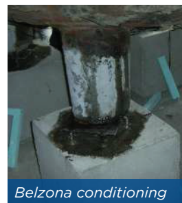
Belzona being applied
