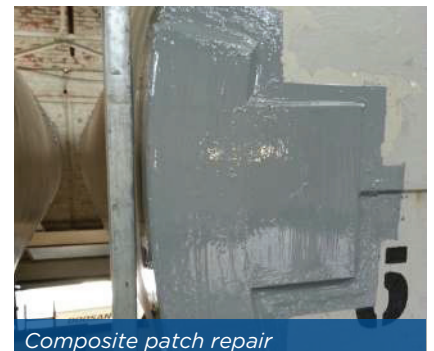
Composite patch repair
