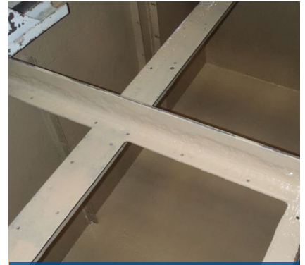
Immersion coating applied
