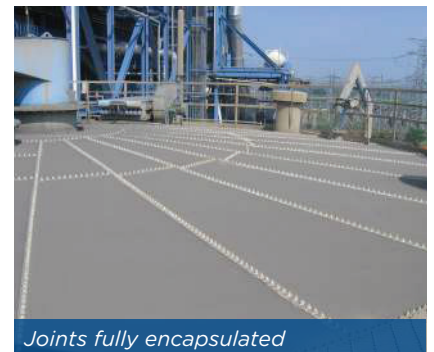
Base sealed with a Belzona coating
