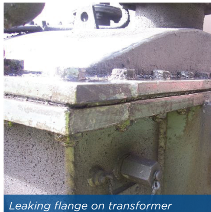
Transformer leaking oil from cracks
