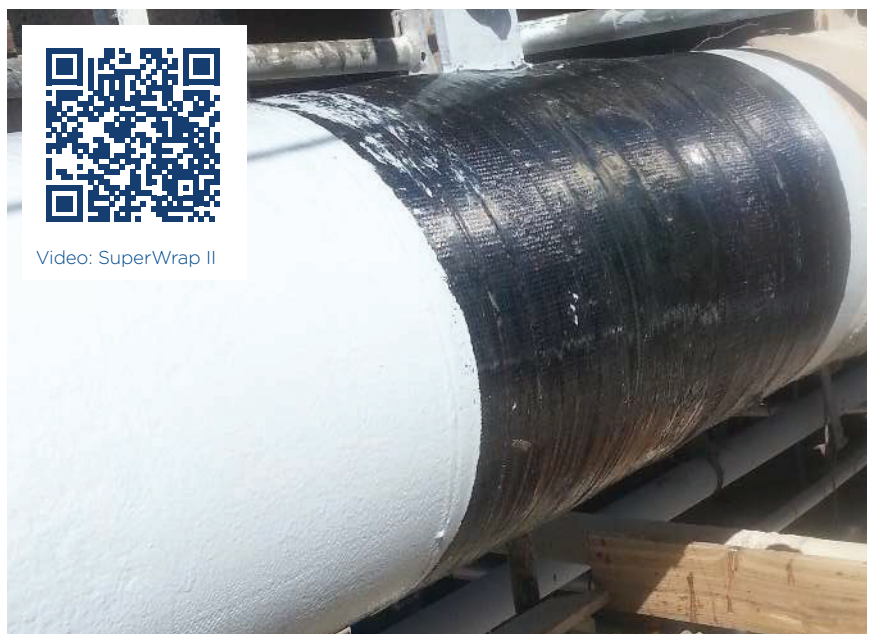
Belzona SuperWrap II compliant to ASME PCC2 Article 4.1 and ISO/TS 24817
