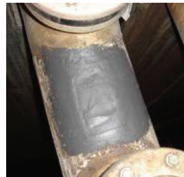
Damaged area repaired
