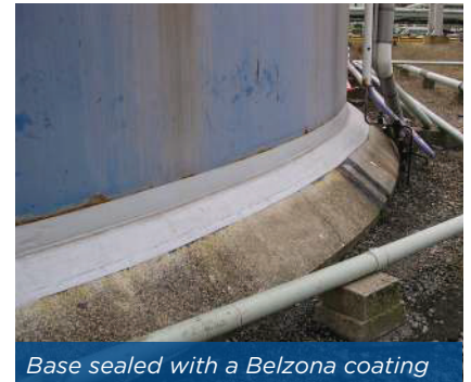
Base sealed with a Belzona coating
