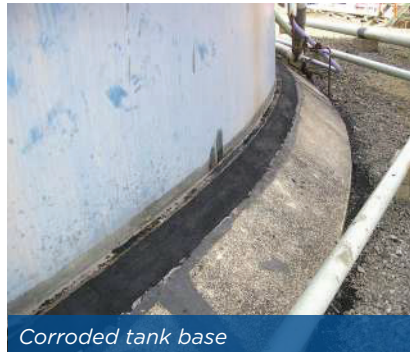
Corroded tank base
