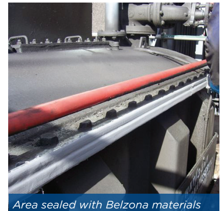
Leak repaired with plate bonding
