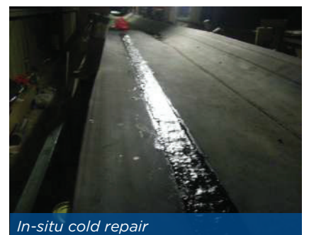
Internal section lined with Belzona
