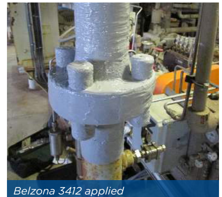
Belzona 3412 applied
