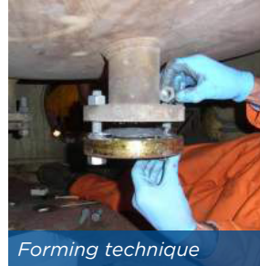
Glass flake lining repair
