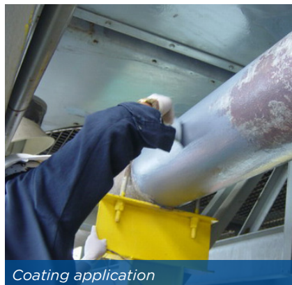
Corrosion under insulation
