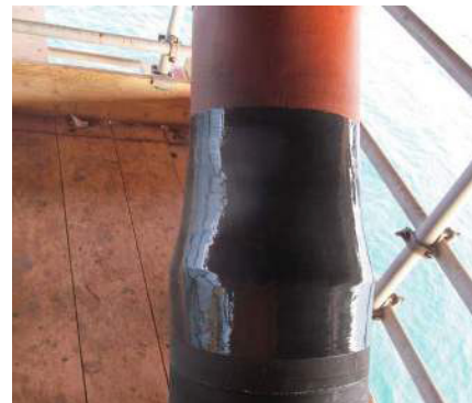
Corrosion repaired and cladding sealed
