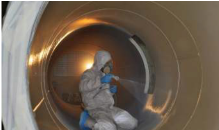
100% solids epoxy protective linings for erosion-corrosion protection
