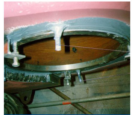
Rudder bearing bonding - bottom view
