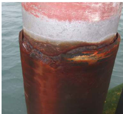
Corroded riser
