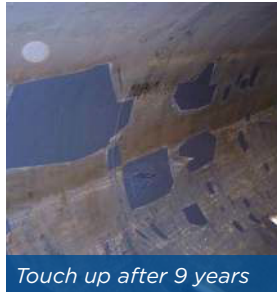
Glass flake lining repair
