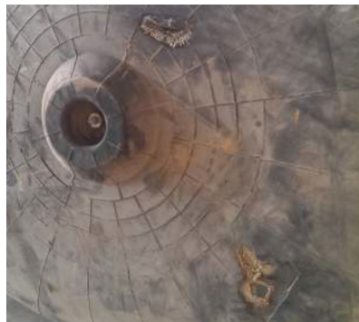
Deteriorated fender
