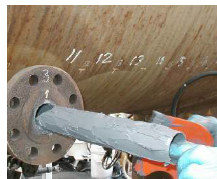
Prefabricated Belzona insert bonded into small bore nozzle
