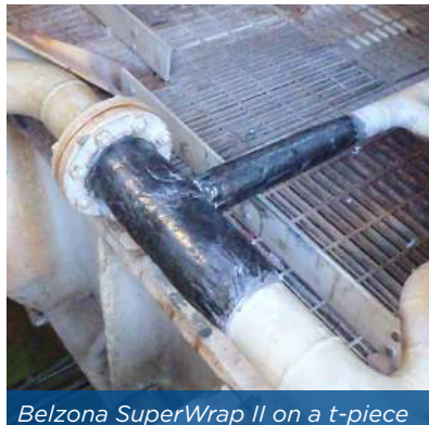
Belzona SuperWrap II on a t-piece
