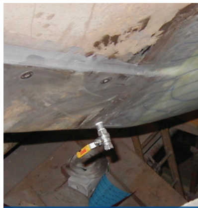
Anchor pocket bonding in progress
