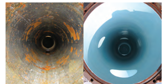
Desulfurization unit protected with coating
