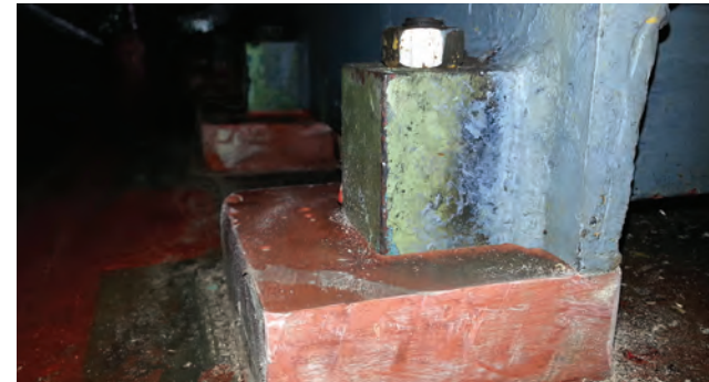
New boiler required chocking into place
