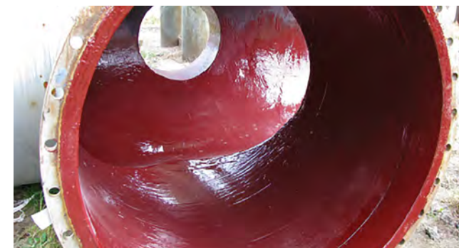
Internal lining protected against chemical attack
