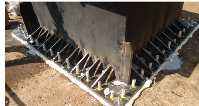
Concrete shimming of crane base
