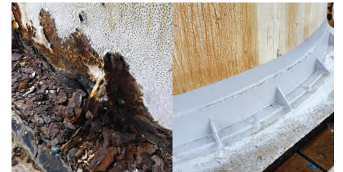
Tank base repaired and restored from corrosion
