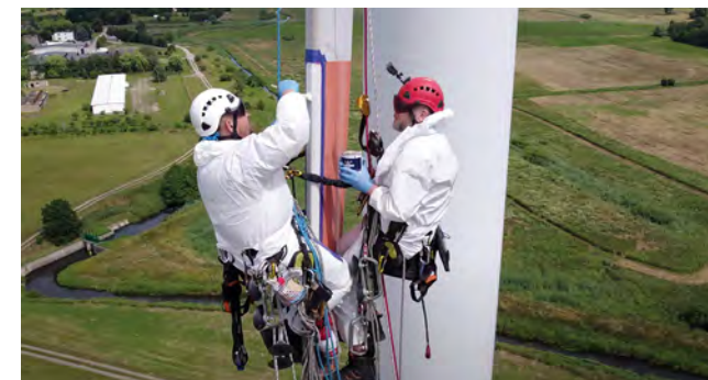
Protection of wind turbine blades
