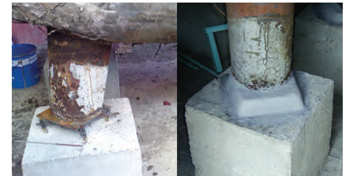
Vessel supports repaired and protected
