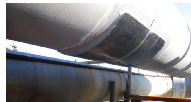
Composite pad installed for pipeline repair
