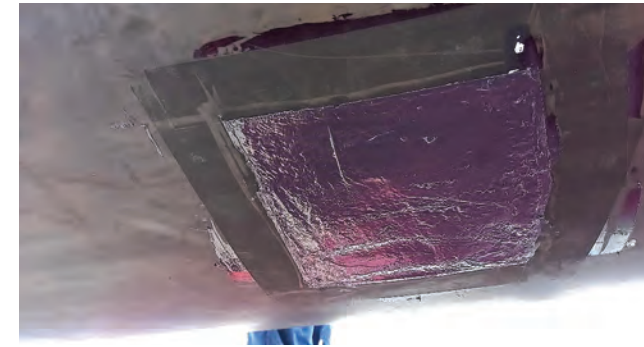
Repaired 4km long conveyor belt back in operation
