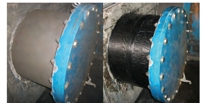
Wrap repair on pipework
