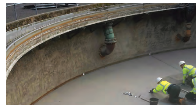
Repair of a large wastewater clarifier suffering erosion and chemical attack
