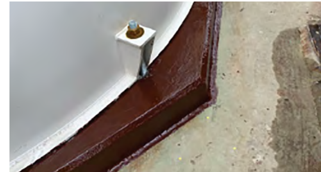
Sulfuric acid tank base protected with Belzona
