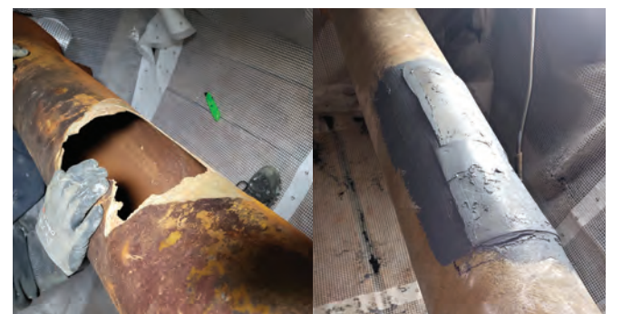
Damaged GRP pipe repaired using Belzona's cold bonding solution
