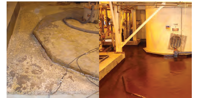
Concrete was rebuilt and protected from sulfuric acid damage
