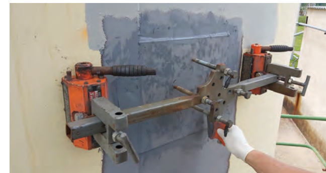
Corroded tank wall repaired
