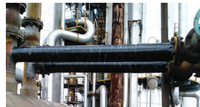
Pipe wall strength restored using compliant pipe wrap
