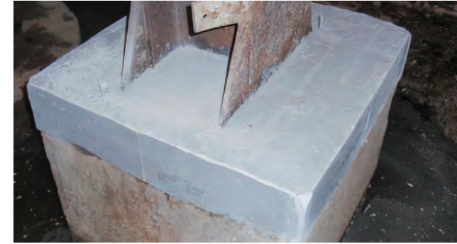
Metallic footing of a pulper and concrete restored
