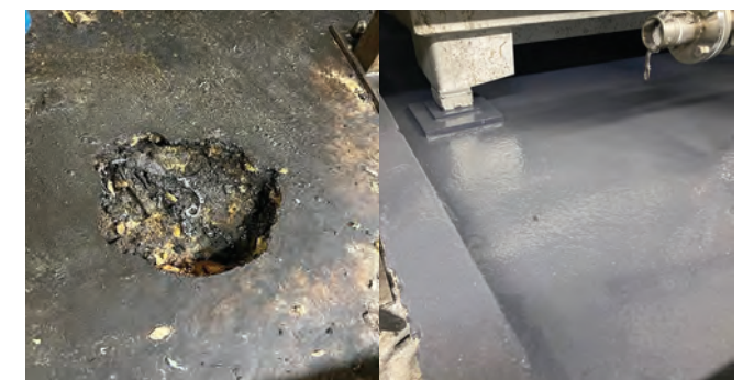
Corroded concrete repaired and protected from chemical attack
