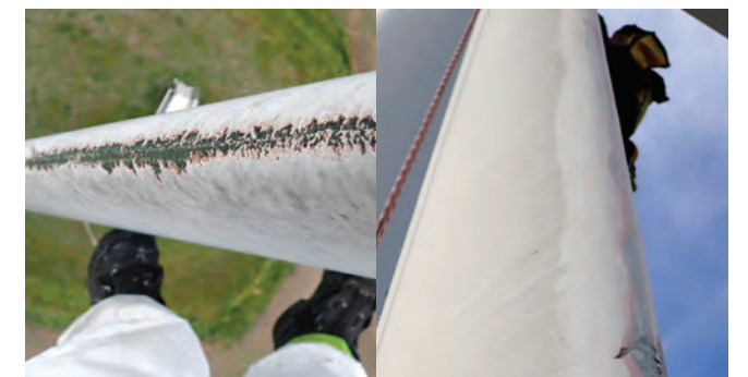
Rain erosion repaired with Belzona leading edge protection solutions
