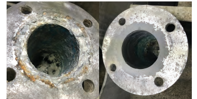
Emergency flange repair
