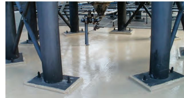
Spirit containment area repaired and protected
