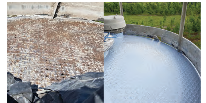
Lid repaired with plate bonding technique
