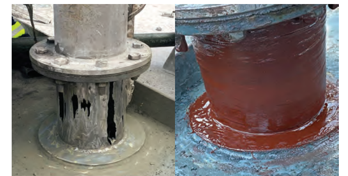
Damaged acid intake nozzle rebuilt
