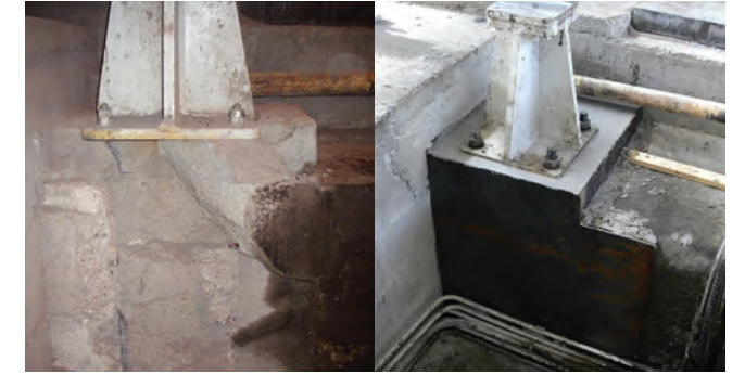
Damaged concrete footing repaired and rebuilt
