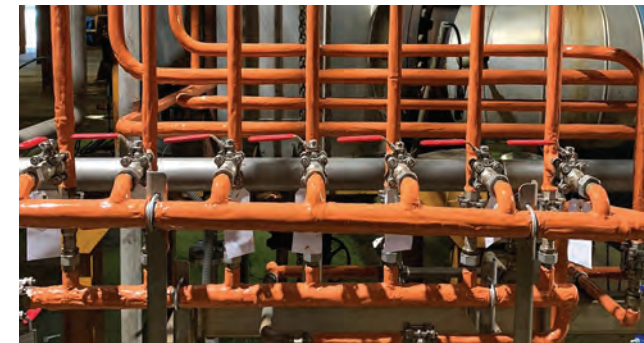
Insulating the thermal process of pipework to reduce heat loss
