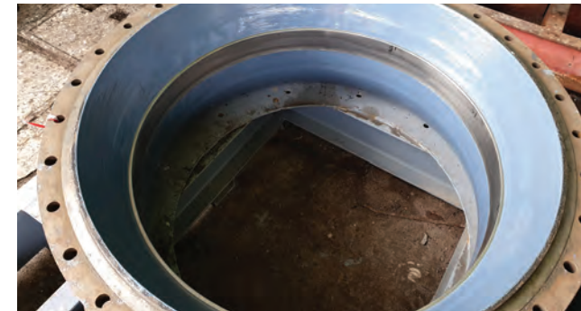
Valve repaired and protected from sea water erosion
